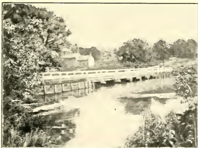
Bridge over Hop Brook and mill pond on the road between Marlboro and Brick Church.
